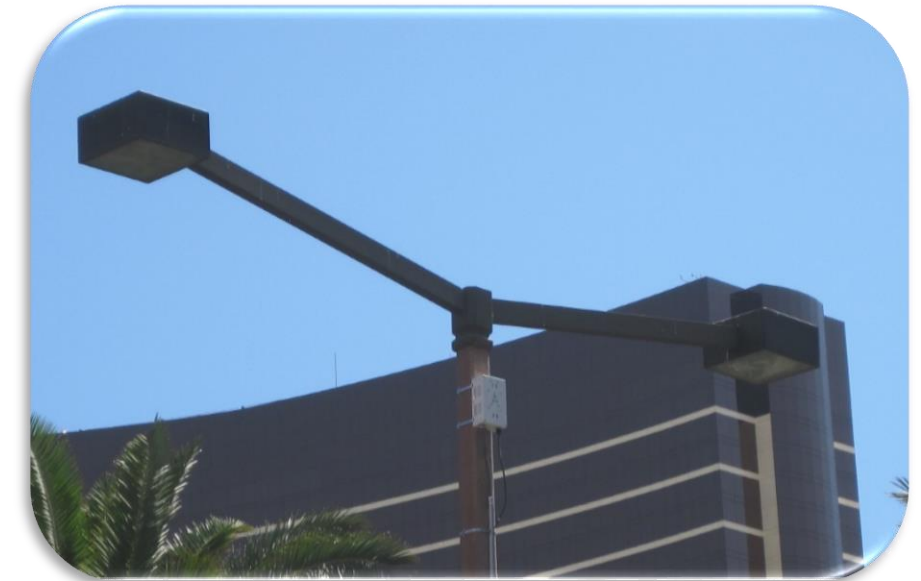
Picture 2.5 – Replaced Pedestrian Lighting - 2012.
