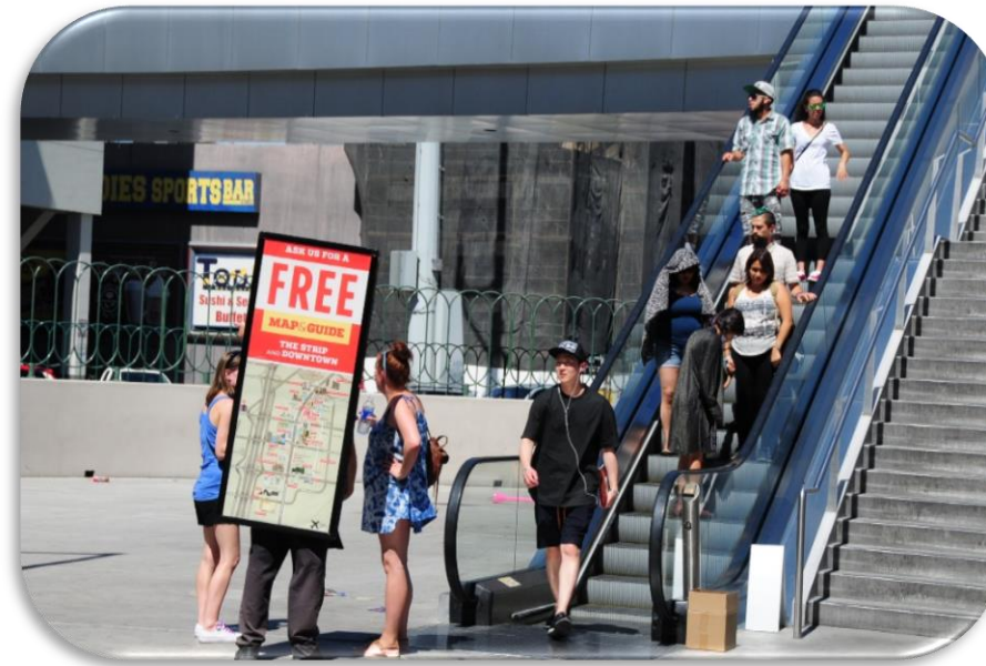
Picture 2.27 – Non-Permanent Obstruction in Escalator Clearance Zone.
