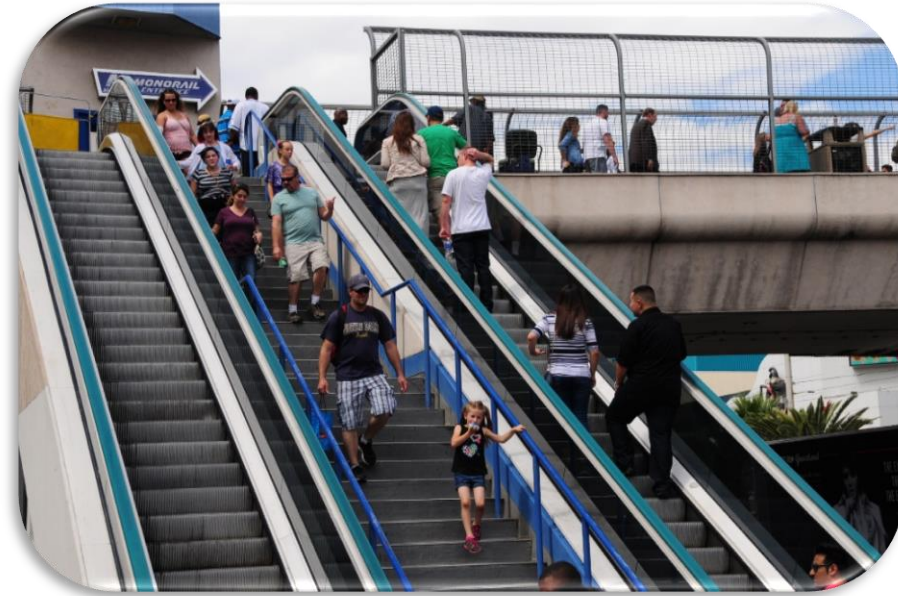
Picture 5.13 – Downward Escalator under Repair.
