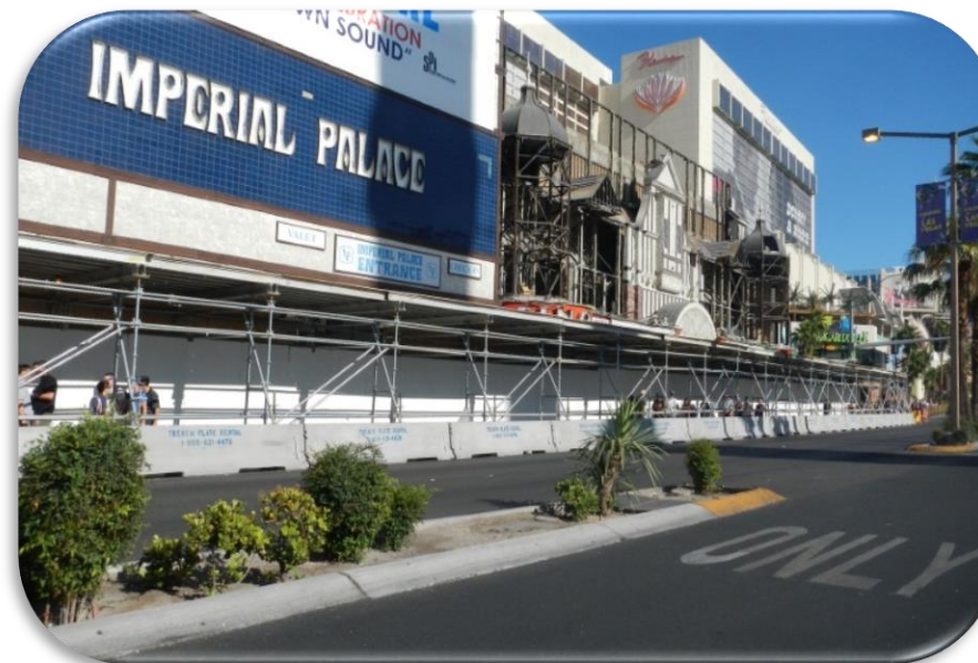
Picture 2.2 – Caesars LINQ Construction – 2012.
