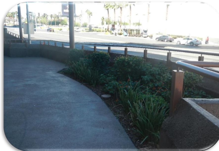
Picture 2.53 – Reconstructed Containment along New CVS Store at Treasure Island.
