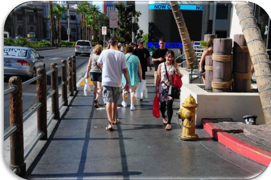
Picture 2.7 – Typical Fire Hydrant at Margaritaville - 2012.
