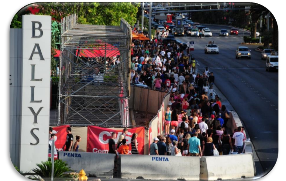
Picture 5.17 – Work Zone Walkway on Memorial Day Weekend 2015.
