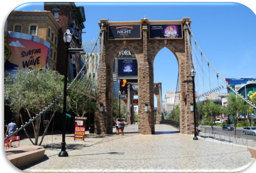
Picture 4.3 – New York-New York Bridge.
