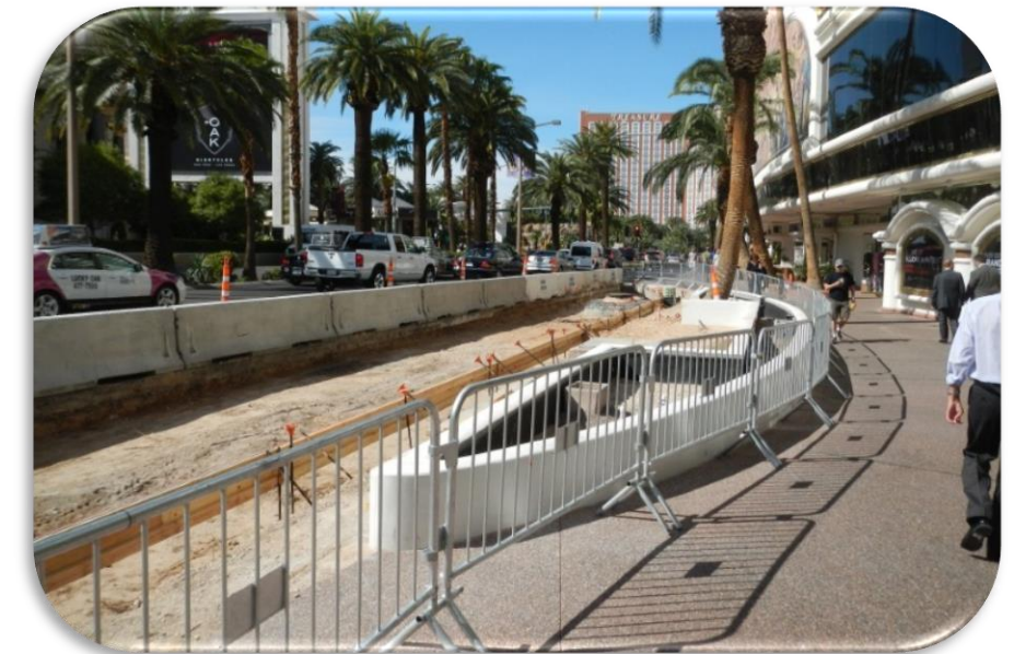
Picture 2.3 – Bus Turnout Construction at Harrah's - 2012.
